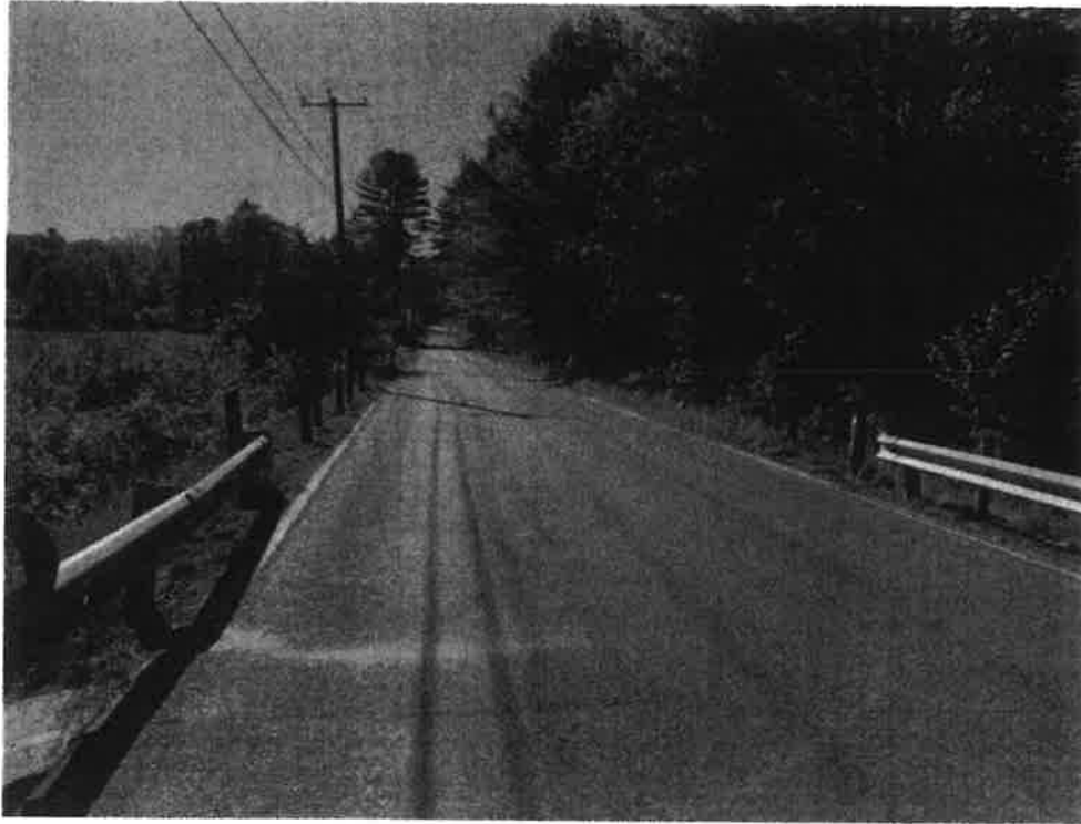
Photo 1 - East Approach to Bridge (Facing West)
