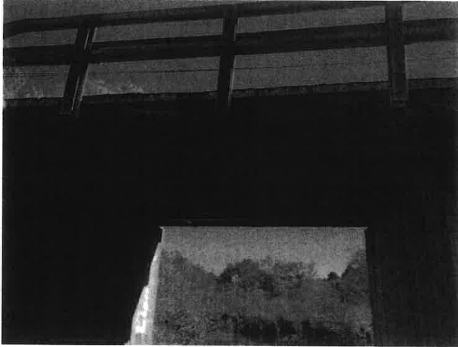
Photo 9 – Downstream Face (Looking Upstream)
