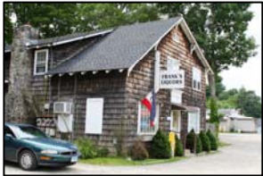
Store with apartment above
